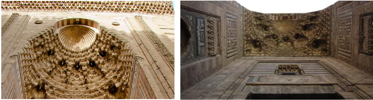
Figure15 a: The upper part of the portal decorated with fractal muqarnas and fractal half dome structure shape.
